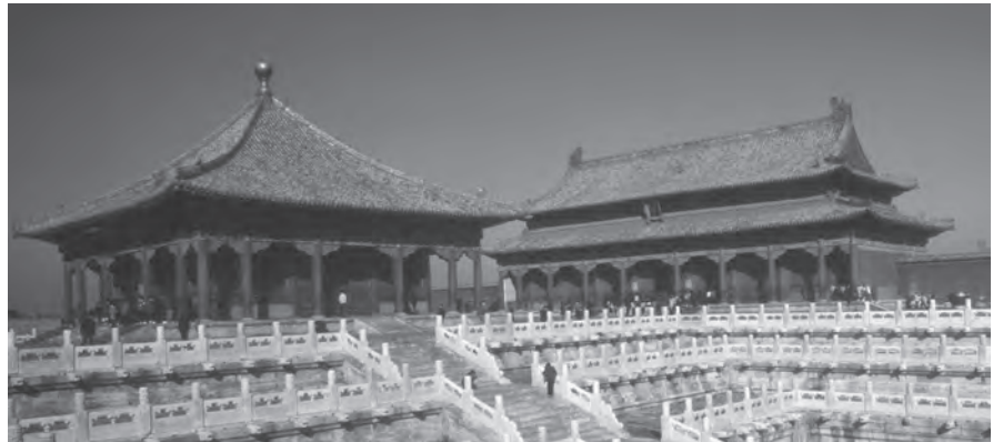
Note the hip roof on the Hall of Middle Harmony (left) and the hipped gable roof on the Hall of Preserved Harmony (right). Source: Wikimedia Commons at http://tinyurl.com/z7z98m9 .
