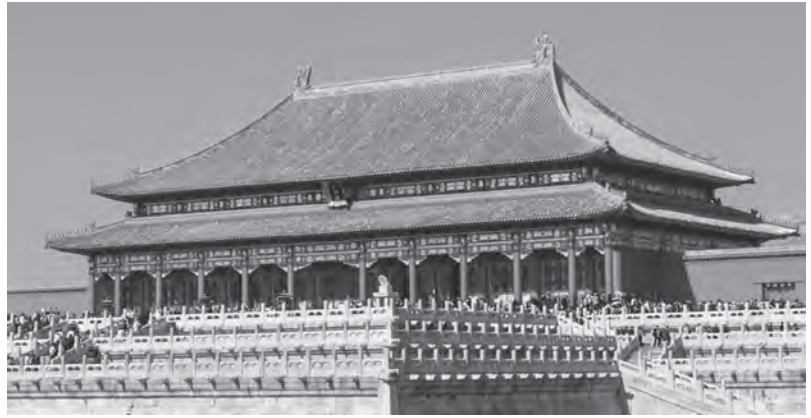
The double-eave hip roof of the Hall of Supreme Harmony. Source: Wikimedia Commons at http://tinyurl.com/zkzws7x .
